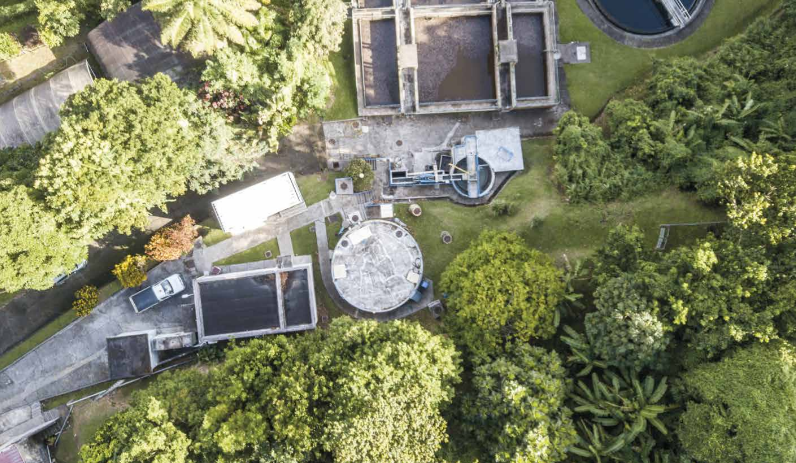
Station d'épuration Godissard Fort-de-France
